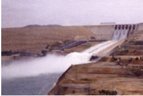
The Keban Dam, Eastern Turkey Breaking out of 4 channels each 6.5m wide across spillways of dam.
